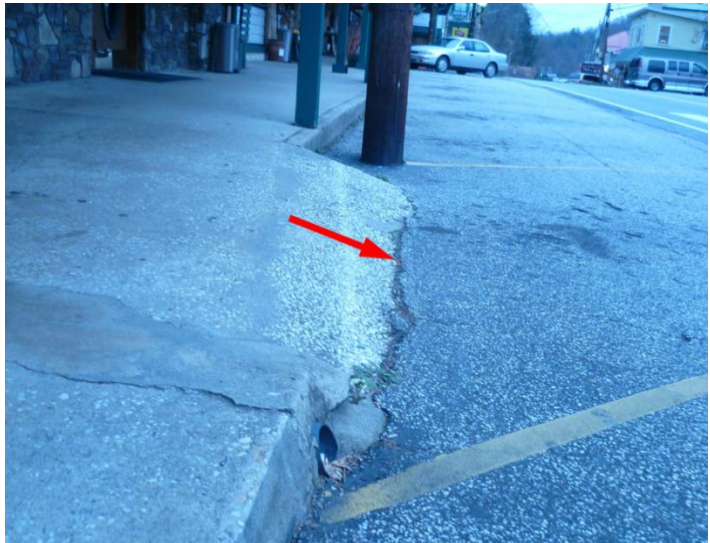
These ramps exceed the 12:1 maximum slope
