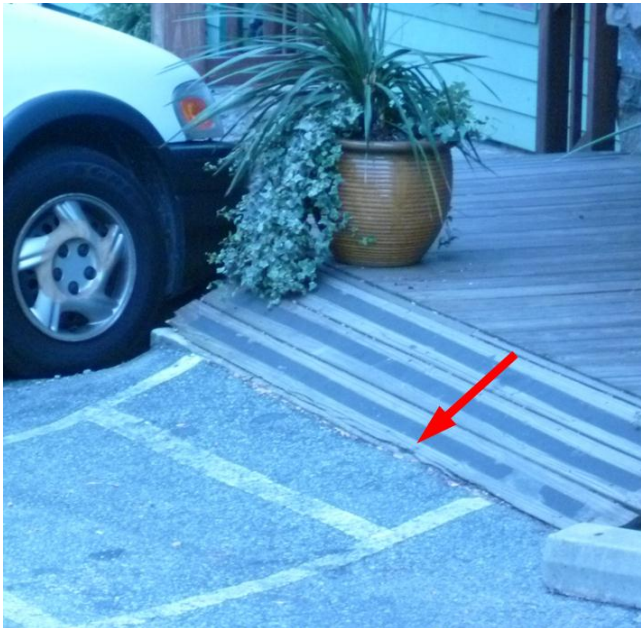
These ramps exceed the 12:1 maximum slope
